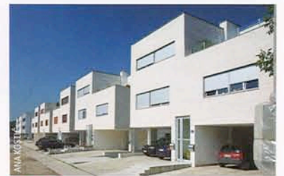
21 FIVE RESIDENTIAL BLOCKS (2009) Architect: Jovan Sarić and Ružica Sarić Address: Dragiše Lapčevića 22
