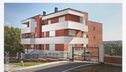
24 TWO RESIDENTIAL BUILDINGS (2010) Architect: Milan Vujović Address: Pivljanina Baja 2. deo 13 and 13a
