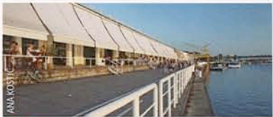
5 CONCRETE HALL (2006) Architect: Aleksandar D. Rodić Address: Karadardeva 2–4
